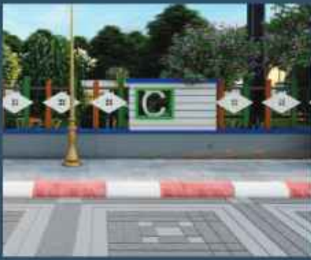
Park Boundary Wall
