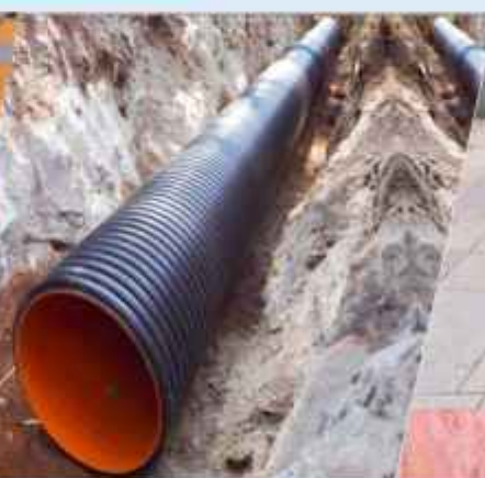
Underground Sewer Pipe Line
