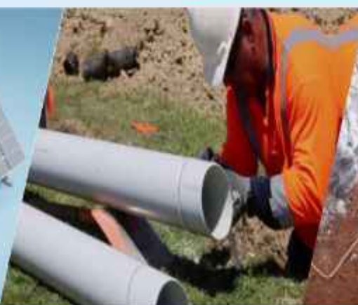
Underground Water Supply Pipe Line
