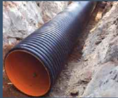
Underground Sewer Pipeline
